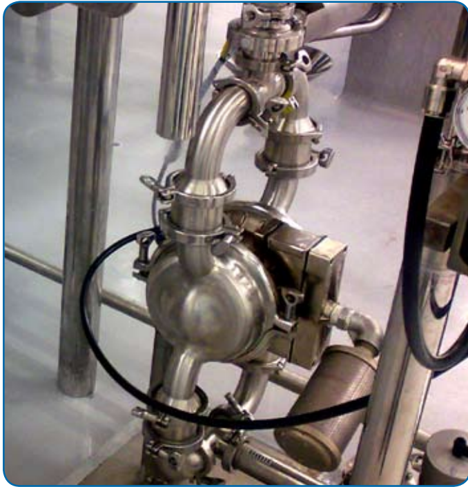
Wilden AODD pump and dampener used in a health care process application.
